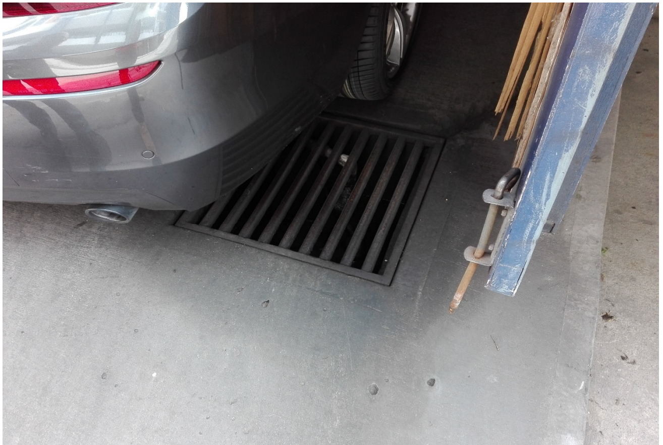
Plate 6: Rinse trap of the oil separator located at 31 Atchison Street.
