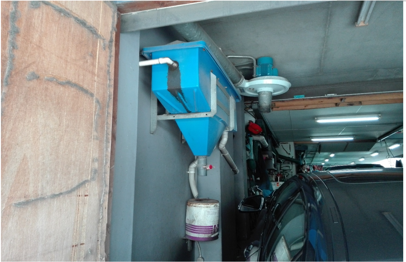
Plate 7: Oil separator AST located at 31 Atchison Street.
